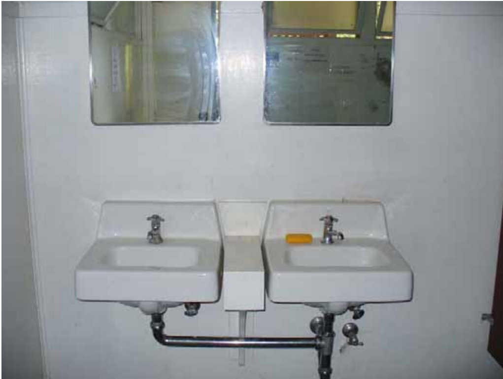
Photo K-2-13. Sinks inside of wood bathroom. (9/04/08)
