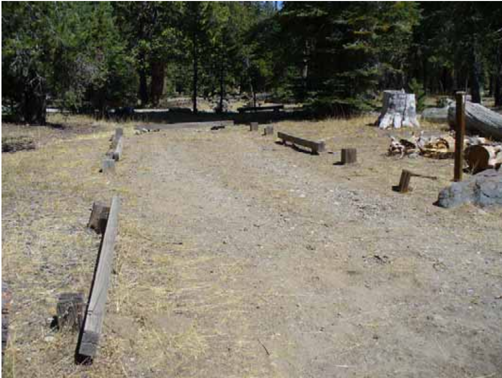
Photo I-2-5. Typical parking spur delineated with wood posts and barriers. Note native surface. (9/4/08)
