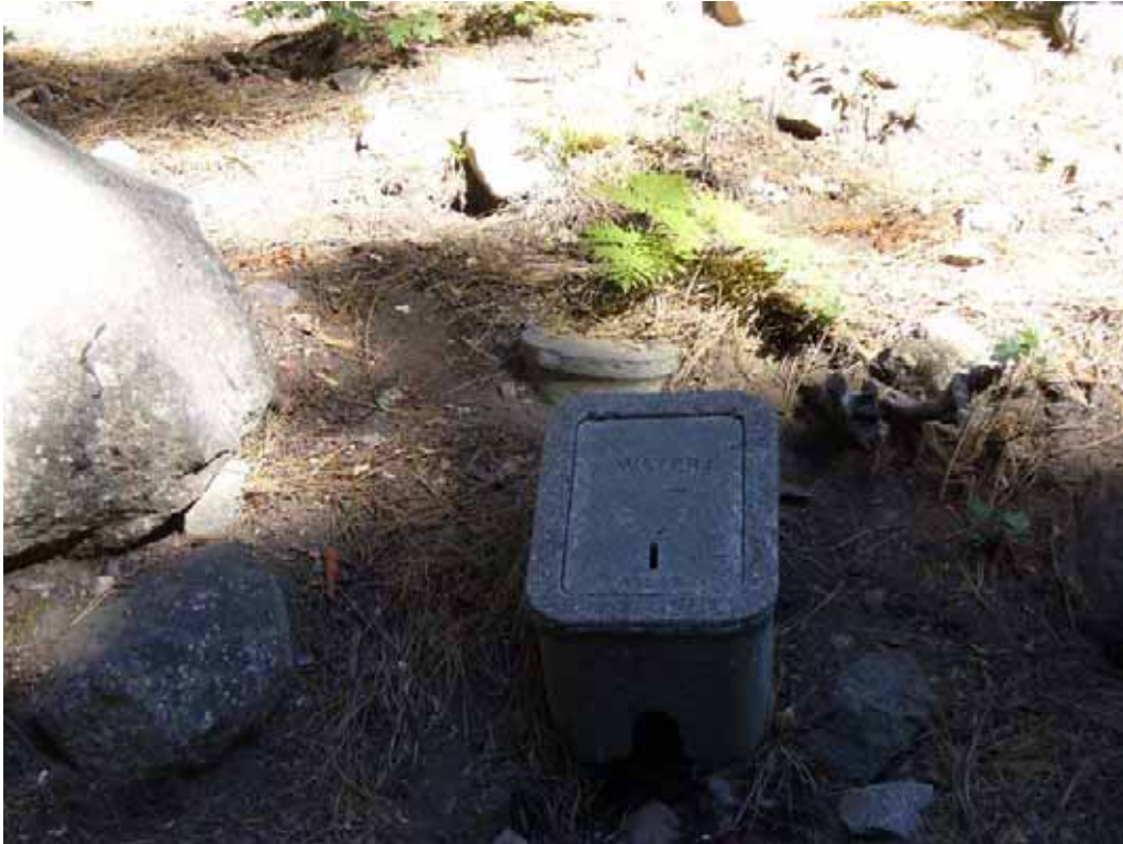
Photo E-2-8. Water valve box on northwest side of parking area. (8/21/08)
