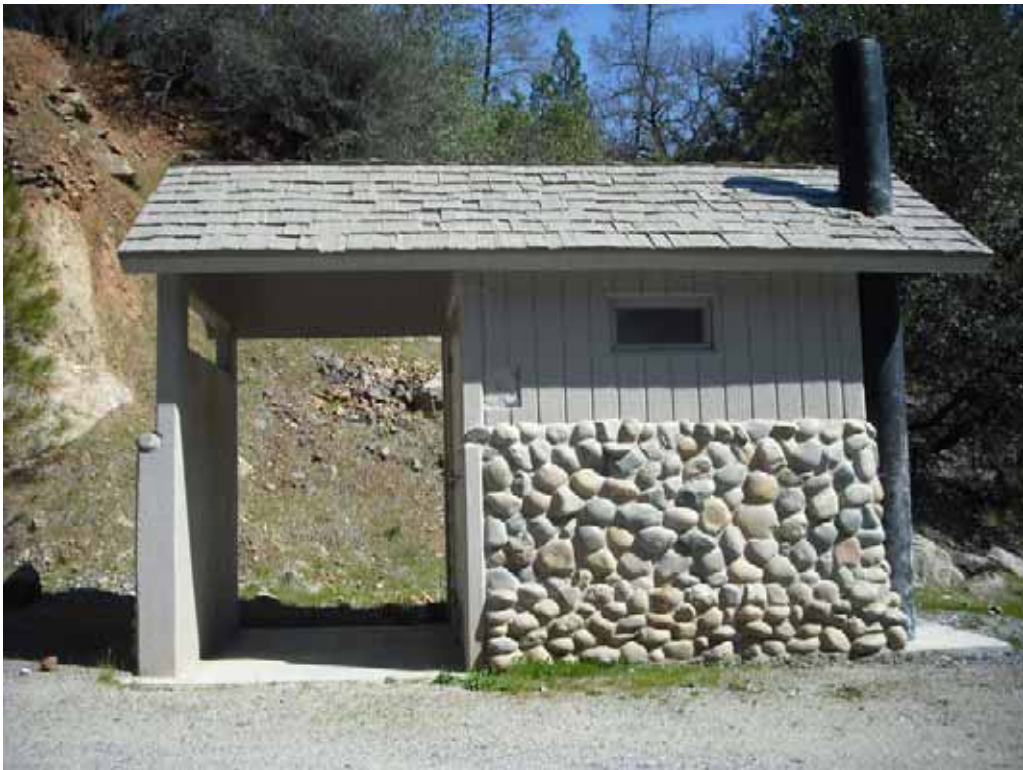
Photo V-2-10. Vault bathroom in good condition located in the Southeast Parking Area. (3/12/09)
