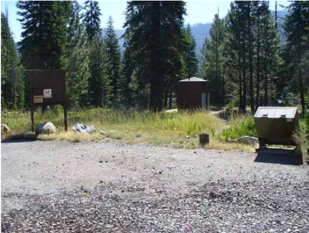
Photo Q-2-9. Entrance of trail to McGuire Beach as viewed from the parking area. Note bear-proof garbage container, information board, and deteriorated asphalt surface. (7/24/08)
