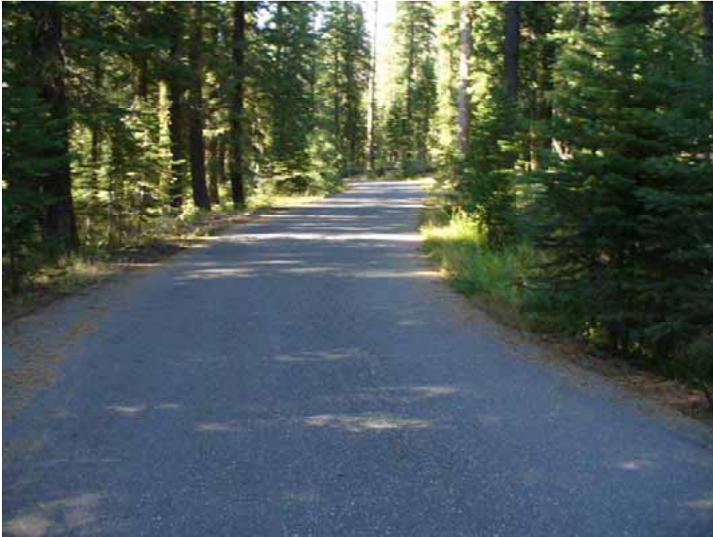
Photo N-2-3. Main access road to Gates Group Campground. (9/4/08)
