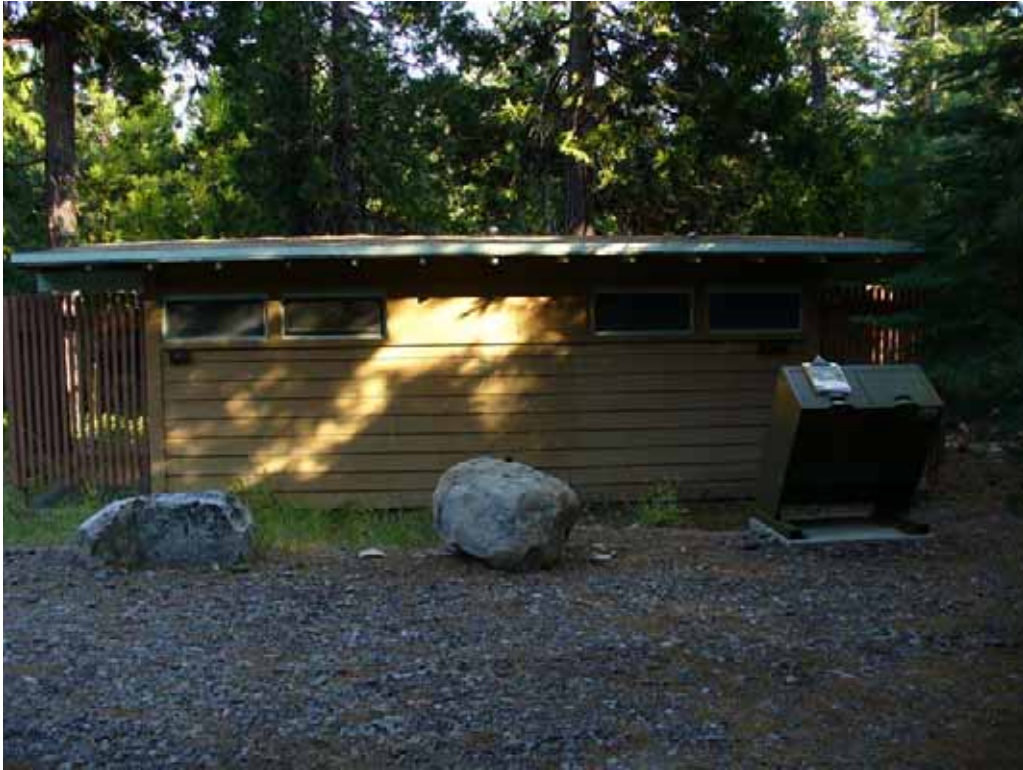
Photo L-2-3. Wood bathrooms with flush toilets and sinks adjacent to Poppy Trailhead parking. Not accessible. (7/23/08)
