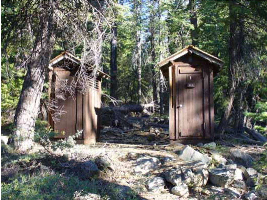
Photo L-2-14. Pit toilets in campground. No accessible. (7/24/08)
