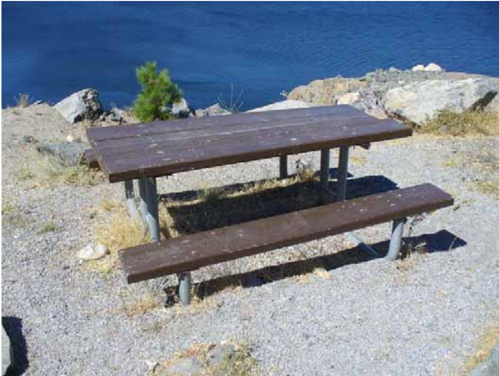
Photo H-2-13. Picnic table located in lower parking lot. Note warped table boards and flaking paint. Not disabled accessible due to design and small obstacles. (8/4/08)
