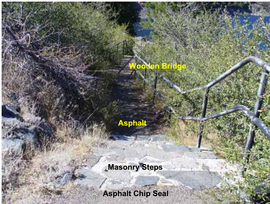
Photo H-2-31. Top portion of trail/stairway to Hell Hole Boat Ramp. Note various surface types: asphalt chip seal landing/masonry steps/asphalt/wooden bridge/asphalt. Also note steel handrails. Not disabled accessible. (8/4/08)
