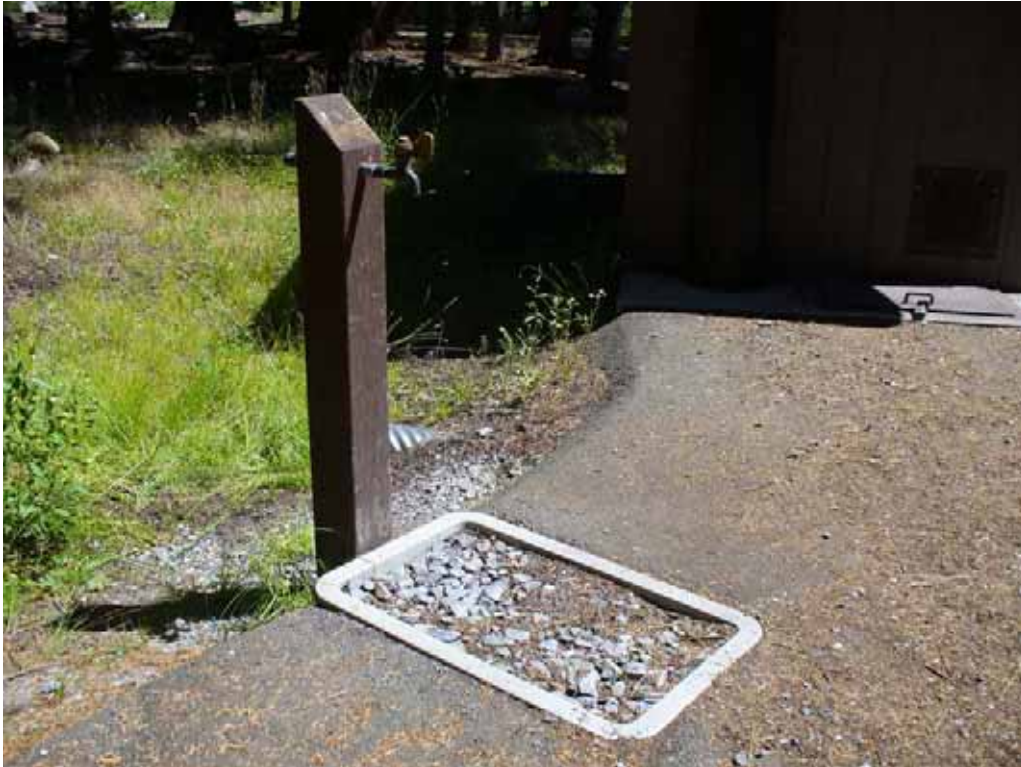
Photo D-2-16. Example water faucet - accessible (8/21/08)
