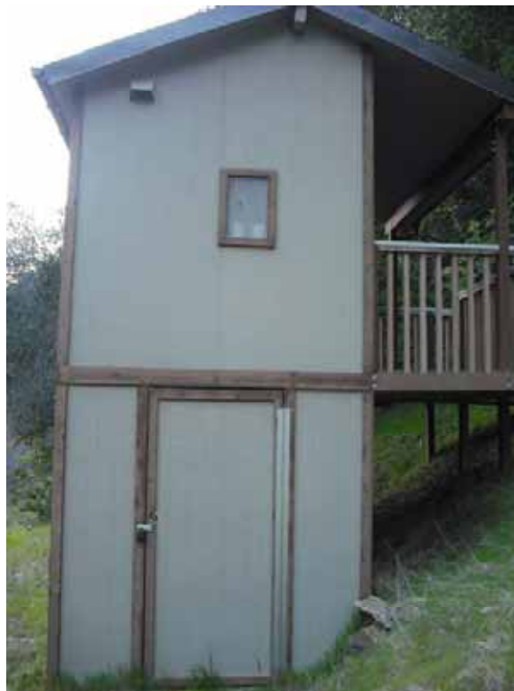
Photo U-2-6. Compost toilet located on the east side of the facility. (3/12/09)
