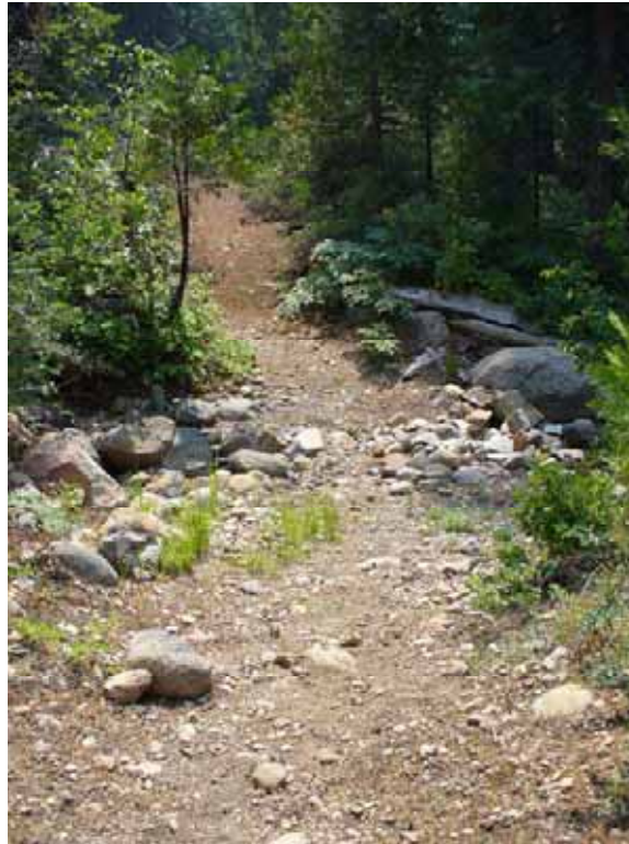
Photo O-2-15. Trail to French Meadows Parking Area. Trail is not considered disable accessible due to obstacles, level changes, excessive slope, and narrow width. (7/23/08)
