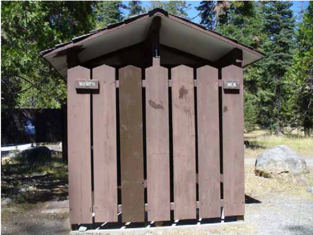
Photo I-2-13. Double-unit, vault toilet building (No. 1). (9/04/08)
