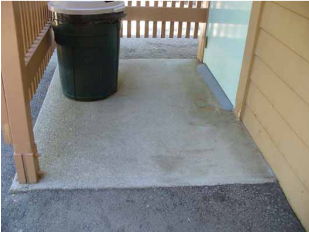
Photo K-2-17. Accessible approach to bathroom. Note the absence of level changes. (9/04/08)
