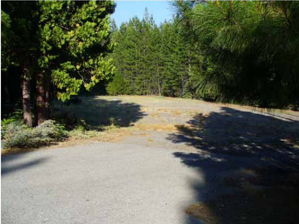
Photo P-2-8. North entrance to McGuire Boat Ramp Parking Area – northeast lot. Note transition from asphalt pavement access road to base rock in parking area. (7/23/08)
