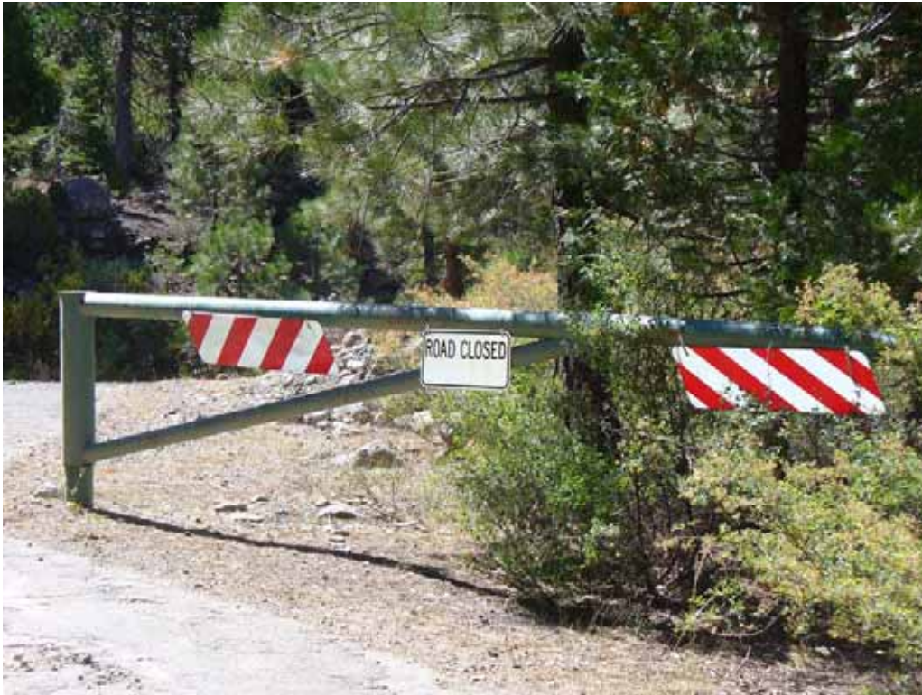
Photo D-2-5. Painted steel swing gate with reflective hazard signs at entrance to Big Meadows Campground. (8/21/09)
