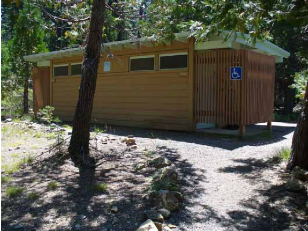
Photo J-2-10. Wood bathrooms with have flush toilets and sinks, converted to be accessible. Note accessible pathway. (7/24/08)
