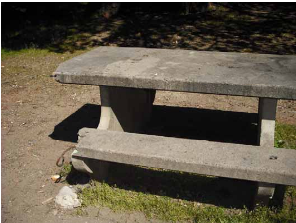
Photo V-2-26. Concrete table located in Campsite 5. Table is damaged and in poor condition. (3/12/09)
