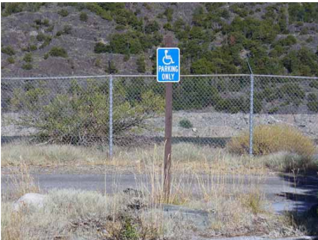
Photo H-2-24. Example of handicap parking sign in parking area. Painted aluminum mounted on wood post. Good condition. (8/4/08)
