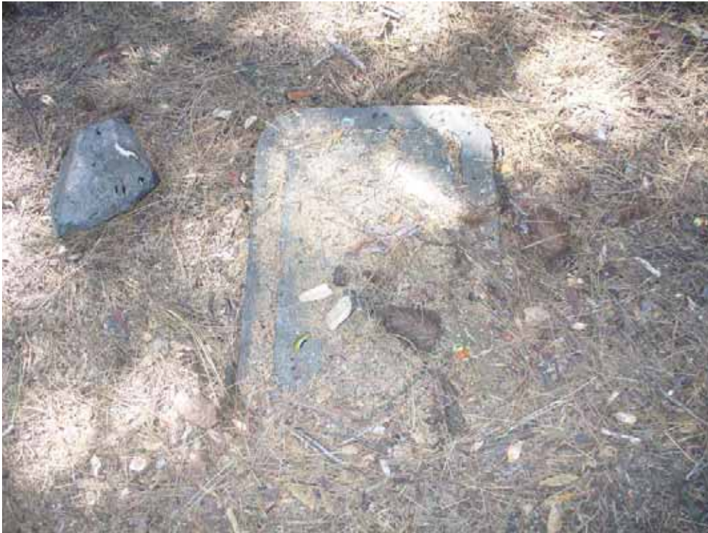
Photo E-2-9. Water valve box on southeast side of parking area. (8/21/08)
