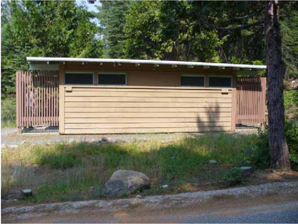
Photo O-2-9. Bathroom located along access road to French Meadows Boat Ramp. This bathroom has flush toilets and sinks but does not meet current USDA-FS condition or accessibility standards. (7/23/08)
