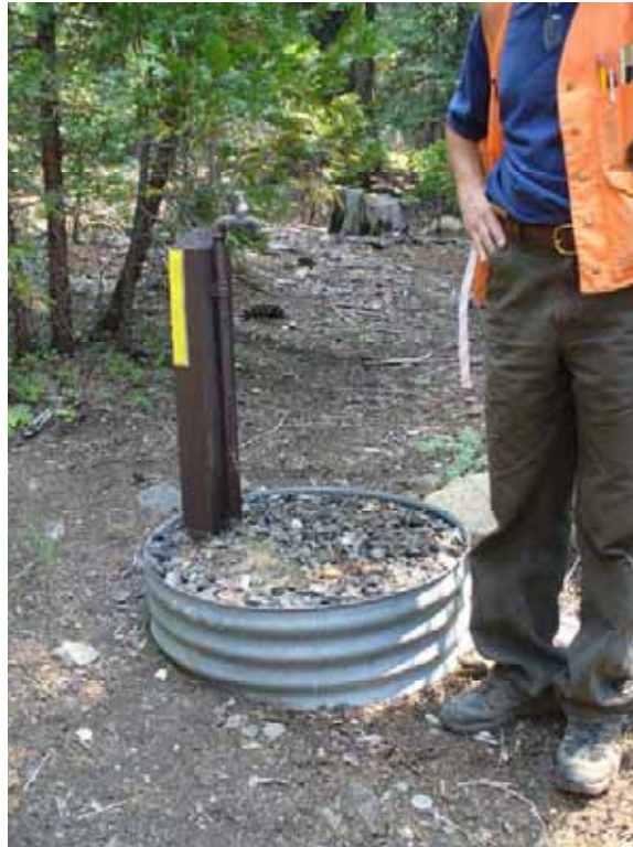
Photo O-2-19. Water faucet in picnic area. Does not meet accessibility standards due to handle design and level changes. (7/23/08)
