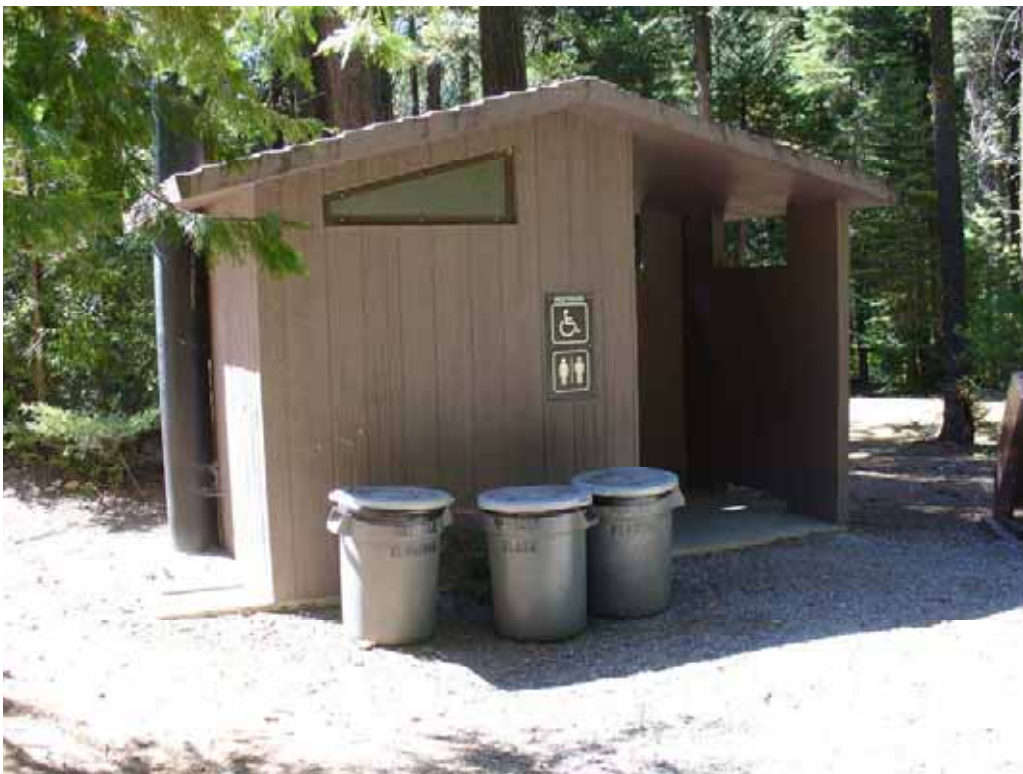
Photo R-2-14. Single unit accessible vault toilet along pathway to Unit 2. (8/21/08)
