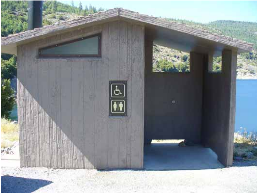
Photo H-2-9. Single unit pre-cast concrete toilet (CXT). Disabled accessible and in good condition. (8/4/08)
