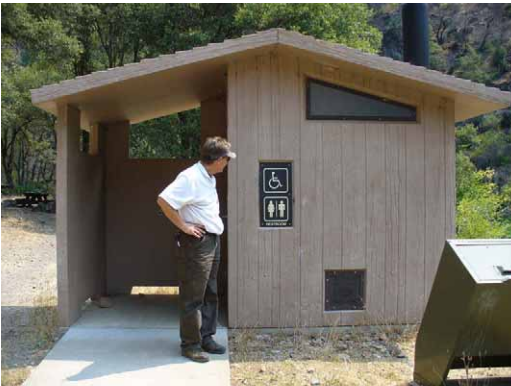
Photo S-2-4. Single unit, pre-fabricated concrete toilet (CXT) at Ralston Picnic Area. (7/23/08)
