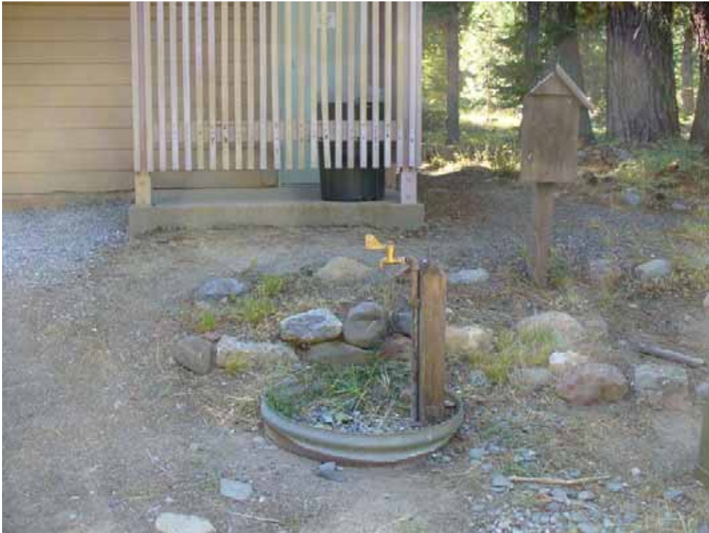
Photo K-2-15. Faucet with accessible handle. (9/04/09)
