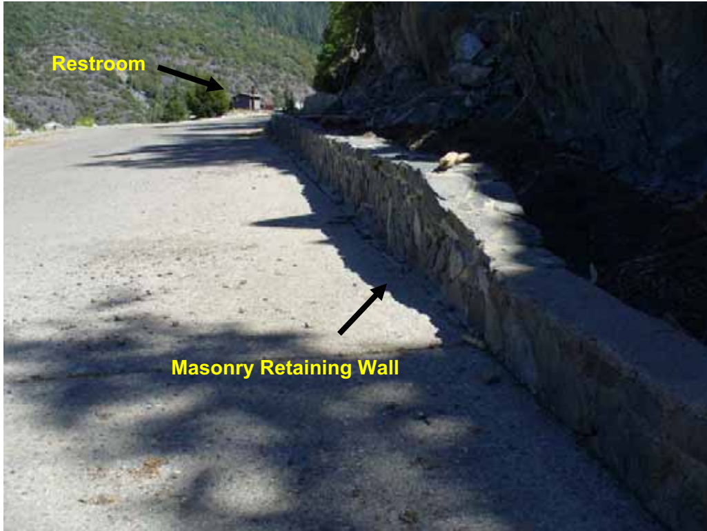
Photo H-2-3. Upper end of Hell Hole Boat Ramp. Note restroom at top of ramp, masonry retaining wall, and concrete surface. (8/4/08)
