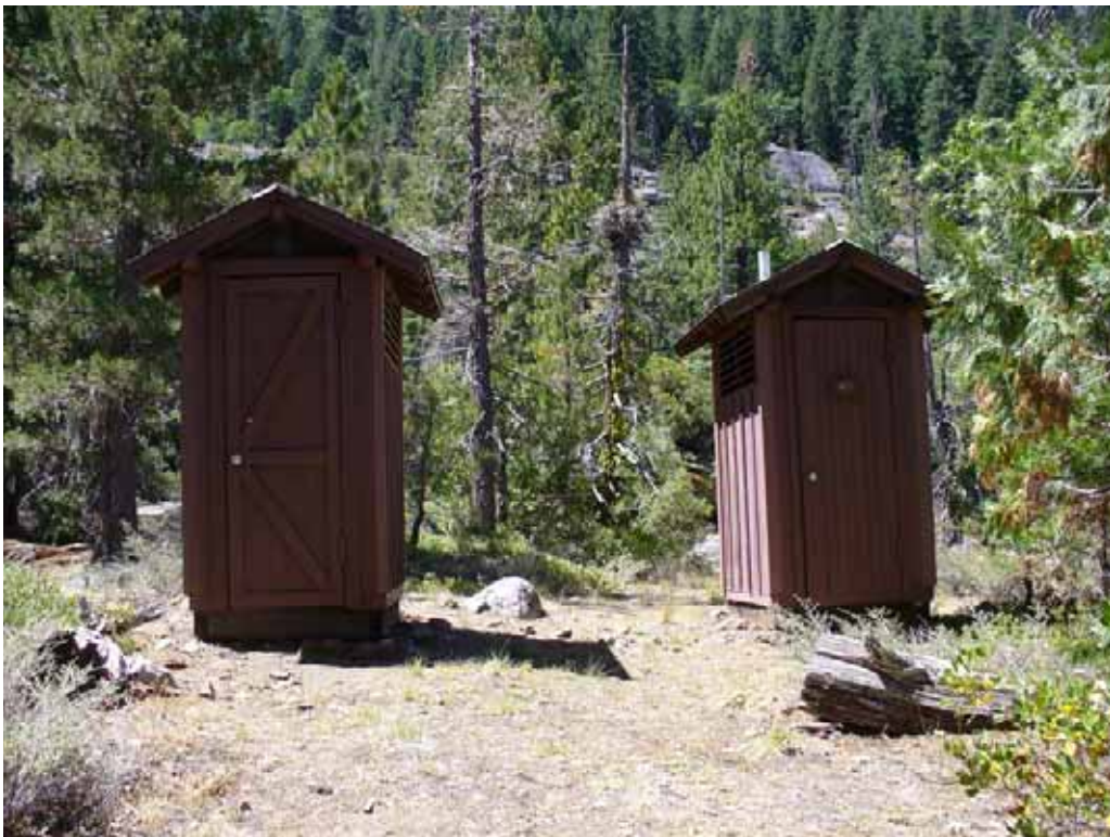
Photo F-2-2. Pit toilets 3 and 4. (8/4/08)
