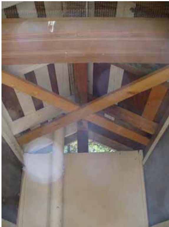
Photo F-2-4. Example of inside of pit toilet. (8/4/08)
