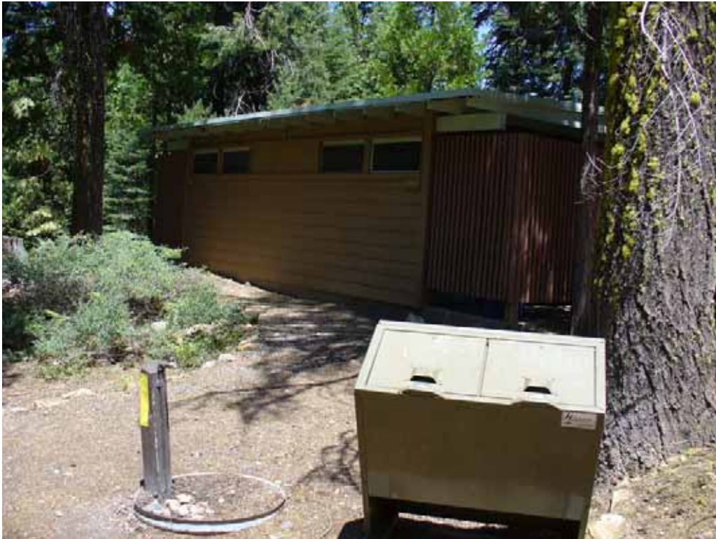
Photo J-2-17. Typical bear-proof garbage container and water faucet. Bathroom #6 in background. (7/24/08)
