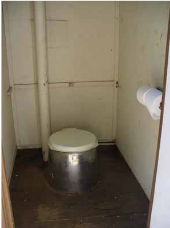
Photo F-2-3. Example of inside of pit toilet. (8/4/08)
