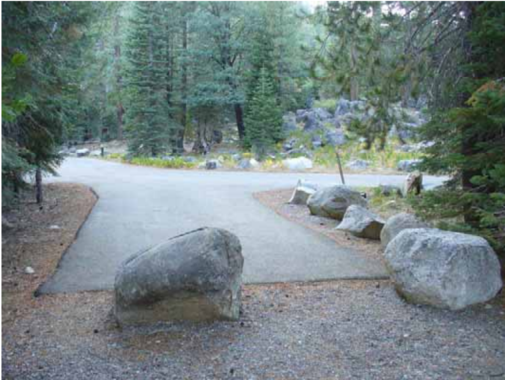
Photo N-2-15. Turn-around area at Lodgepole. Note pavement is in good condition. (9/4/08)
