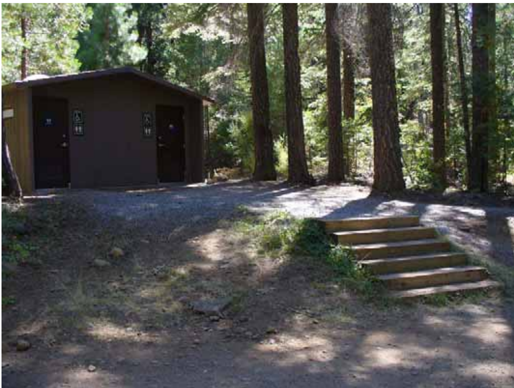
Photo R-2-8. Double unit accessible bathroom with flush toilets located at Unit 1. (8/21/08)
