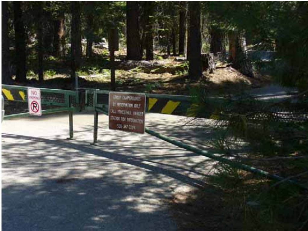
Photo M-2-2. Double swing gate at intersection of FR-96 and Little Wolf and Brush Wolf Main Access Road. This gate is closed and locked when none of the sites are reserved. (7/24/08)
