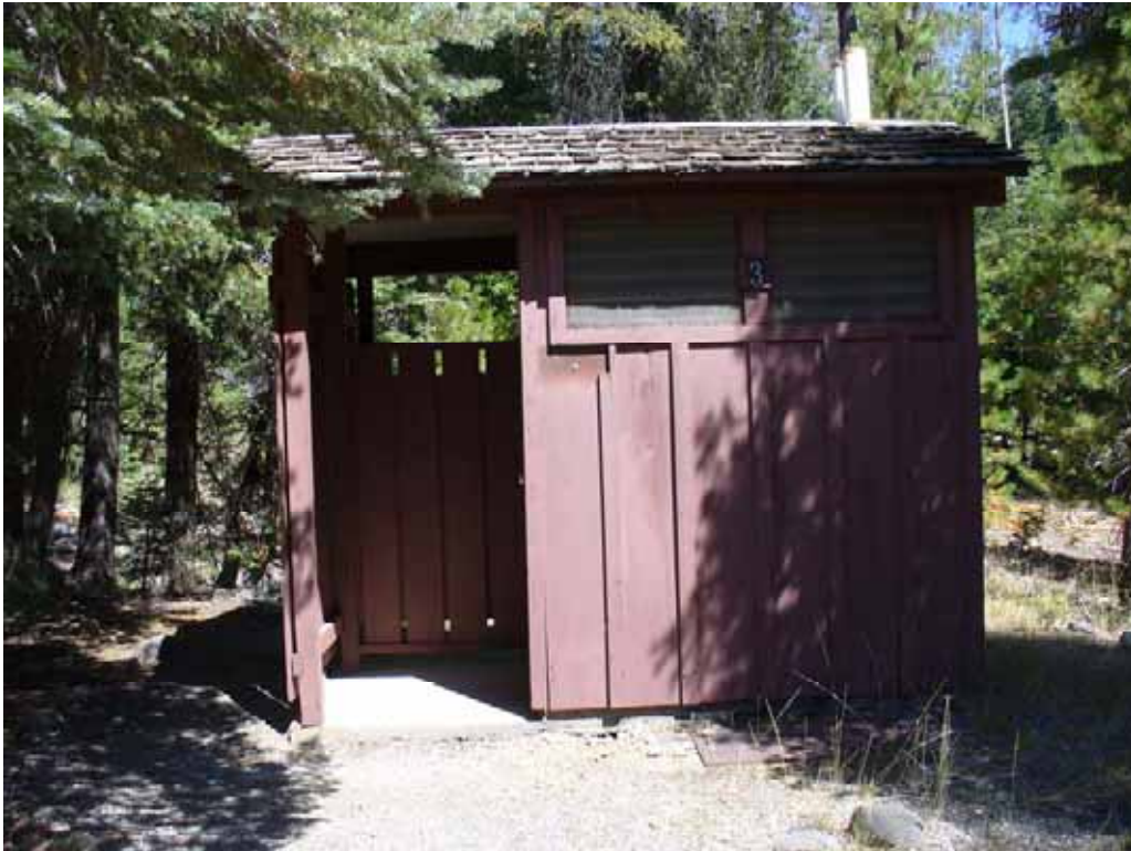
Photo I-2-15. Toilet building No. 3. (9/04/09)
