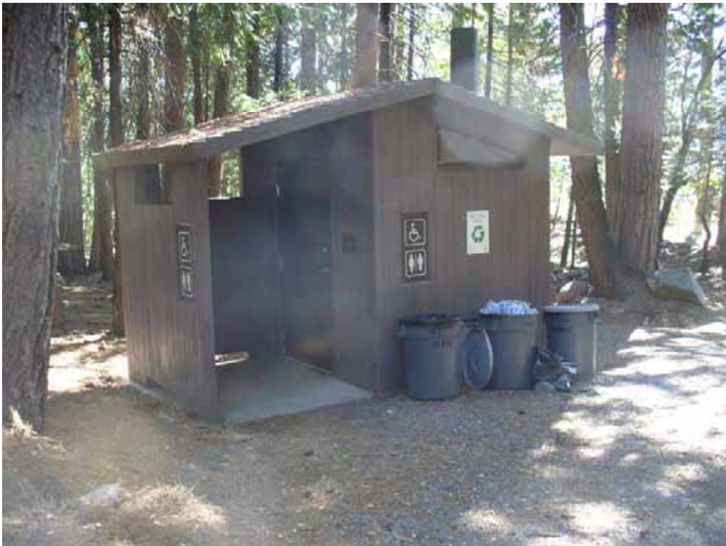
Photo E-2-16. Single-unit, accessible, vault toilet and recycling bins. (8/21/08)
