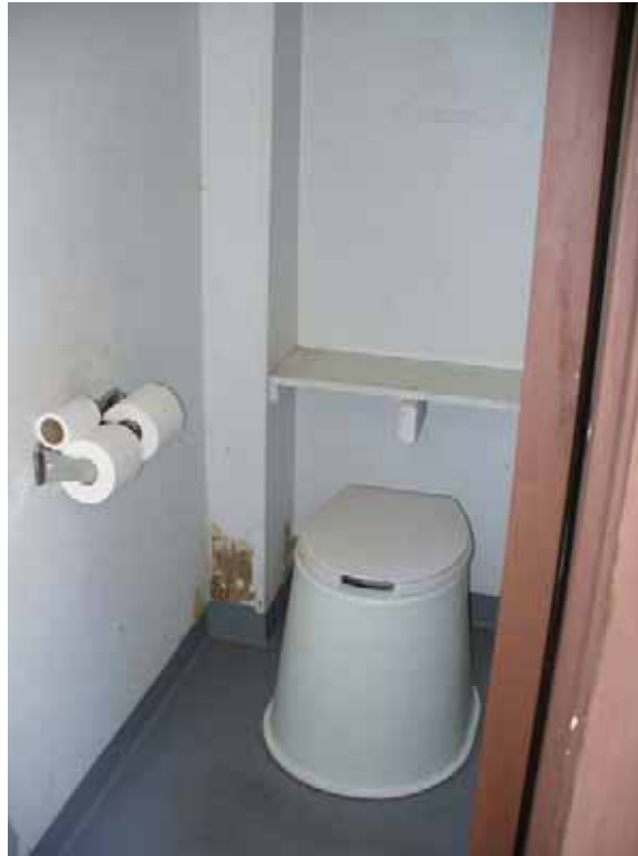
Photo J-2-15. Inside of bathroom #3. (7/24/08)
