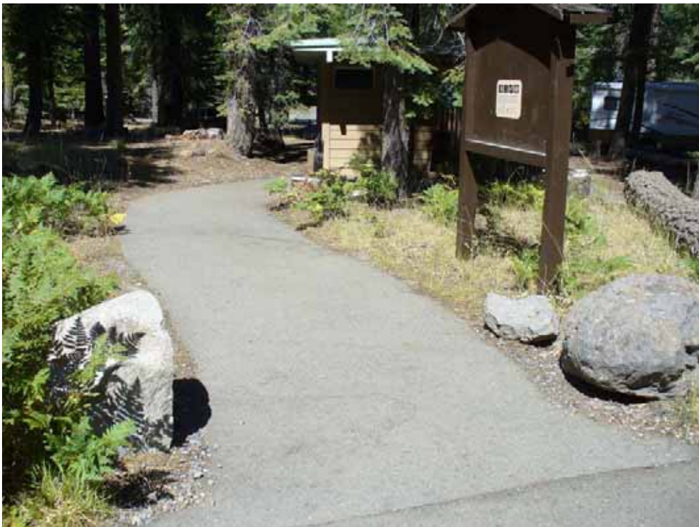
Photo K-2-6. Paved accessible pathway to accessible bathroom with information board, adjacent to host site. All in good condition. (9/04/08).
