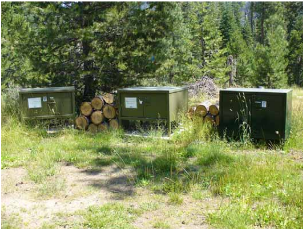
Photo M-2-22. Three bear boxes at Black Bear. Two on concrete pads. Stacked wood was left by fire crews who used this site as a staging area in 2008. Note vegetation. (7/24/08)
