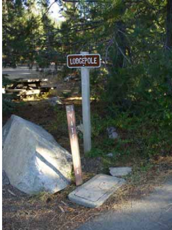
Photo N-2-6. Typical campsite marker and carsonite water line marker. (9/4/08)
