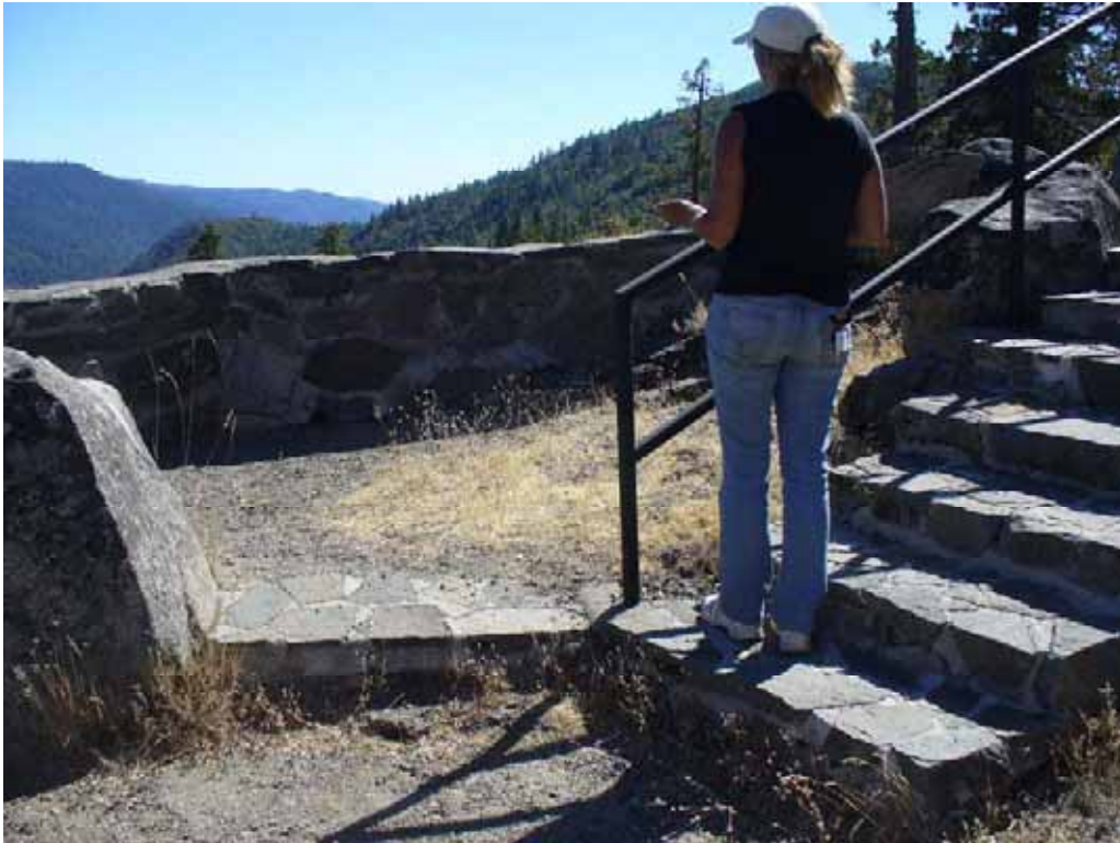
Photo G-2-11. Surface and level changes in Hell Hole Vista. (8/20/08)
