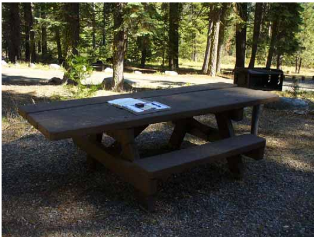
Photo K-2-20. Accessible heavy wood table and pedestal grill at accessible Site 21. Note clear space around table and level, crushed rock surface. (9/04/08)
