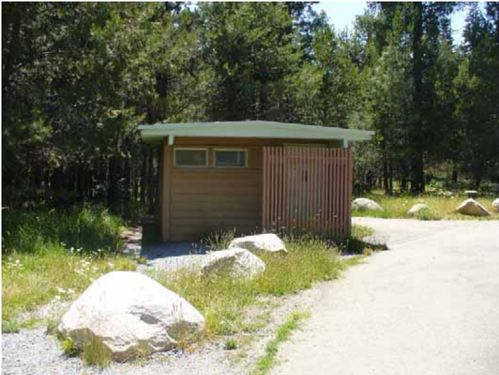
Photo M-2-20. Side view of bathroom at Black Bear from parking area. This bathroom has flush toilets and sinks and was retrofitted to meet accessibility standards. (7/24/08)
