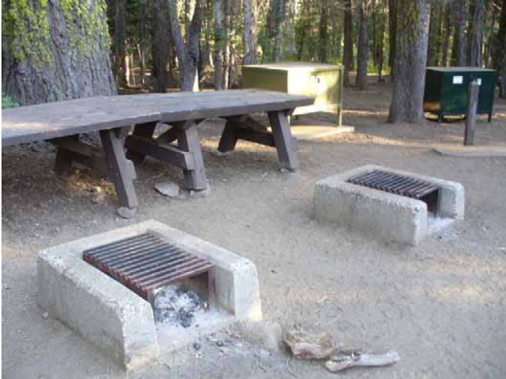
Photo N-2-18. Typical heavy wood serving tables and concrete stoves with steel grills in Gates Group Campground. This photograph was taken at Aspen. (9/4/08)
