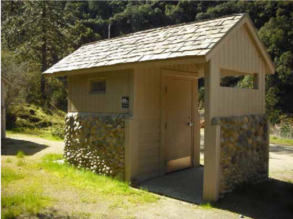
Photo V-2-4. Close-up of bathroom located in Northwest Parking Area. (3/12/09)
