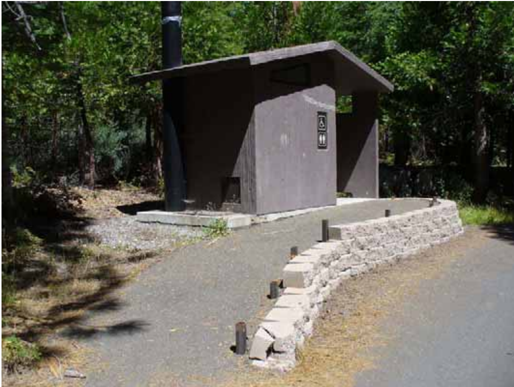
Photo D-2-15. New single-unit, pre-cast concrete toilet (CXT) – accessible. Note that ramp is missing handrail. The handrail was added later in 2008.
