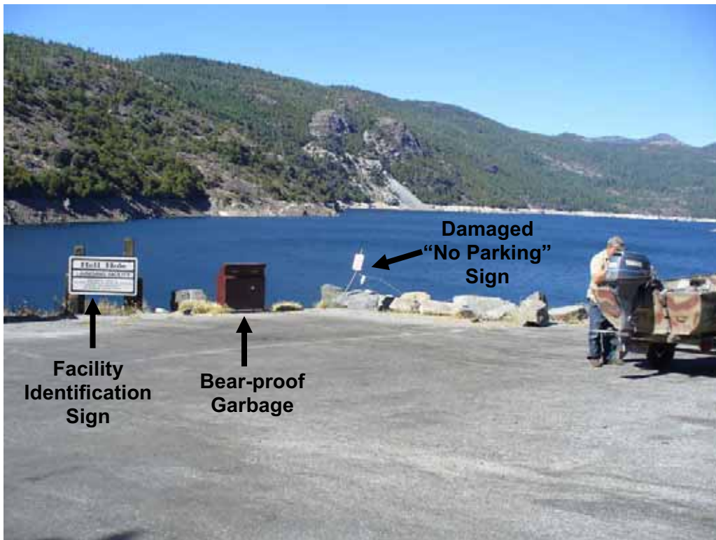
Photo H-2-8. Hell Hole Boat Ramp Parking Area, lower lot. Surface is in good condition but striping has faded. Note facility identification sign, bear-proof garbage container, and damaged "no parking" sign. (8/4/08)
