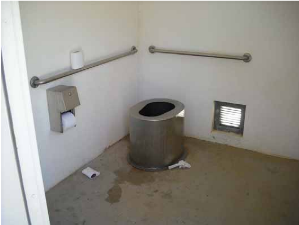
Photo V-2-5. Example interior of bathroom located in the Northwest Parking Area. (3/12/09)
