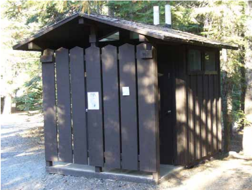
Photo N-2-9. Typical vault bathroom in Gates Group Campground. This bathroom is located in Ponderosa Campground. None of the bathrooms in the Gates Group Campground are accessible. (9/4/08)
