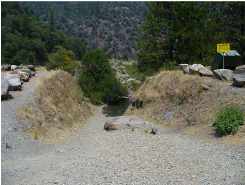
Photo T-2-4. Boat launch ramp. Note warning sign and bear proof garbage to right of ramp. (7/23/08)
