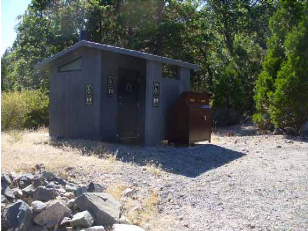
Photo G-2-4. Single-unit vault pre-cast concrete toilet (CXT) and double-bin bear-proof garbage container located in Hell Hole Vista parking area. (8/4/08)
