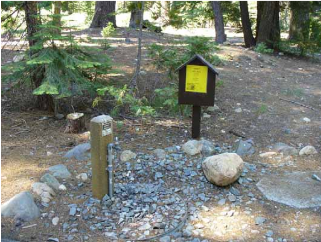
Photo J-2-9. Typical water faucet and information board. Faucet is not accessible. (7/24/08)
