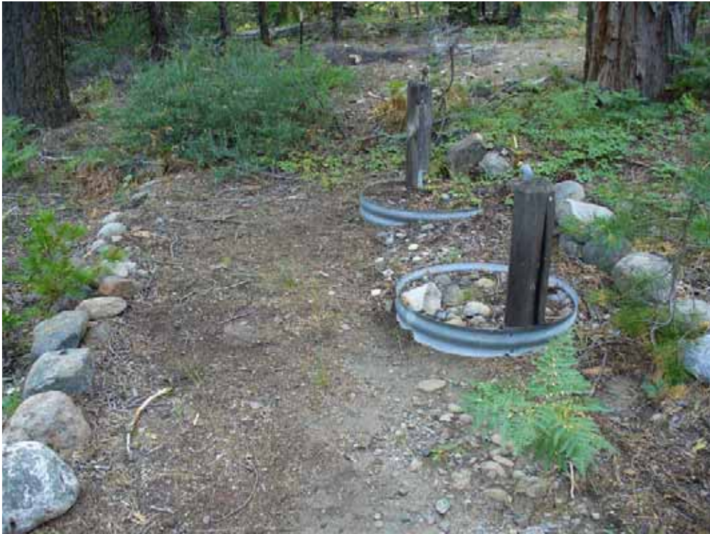
Photo L-2-5. Water faucets behind flush toilets. Not accessible. (7/23/08)
