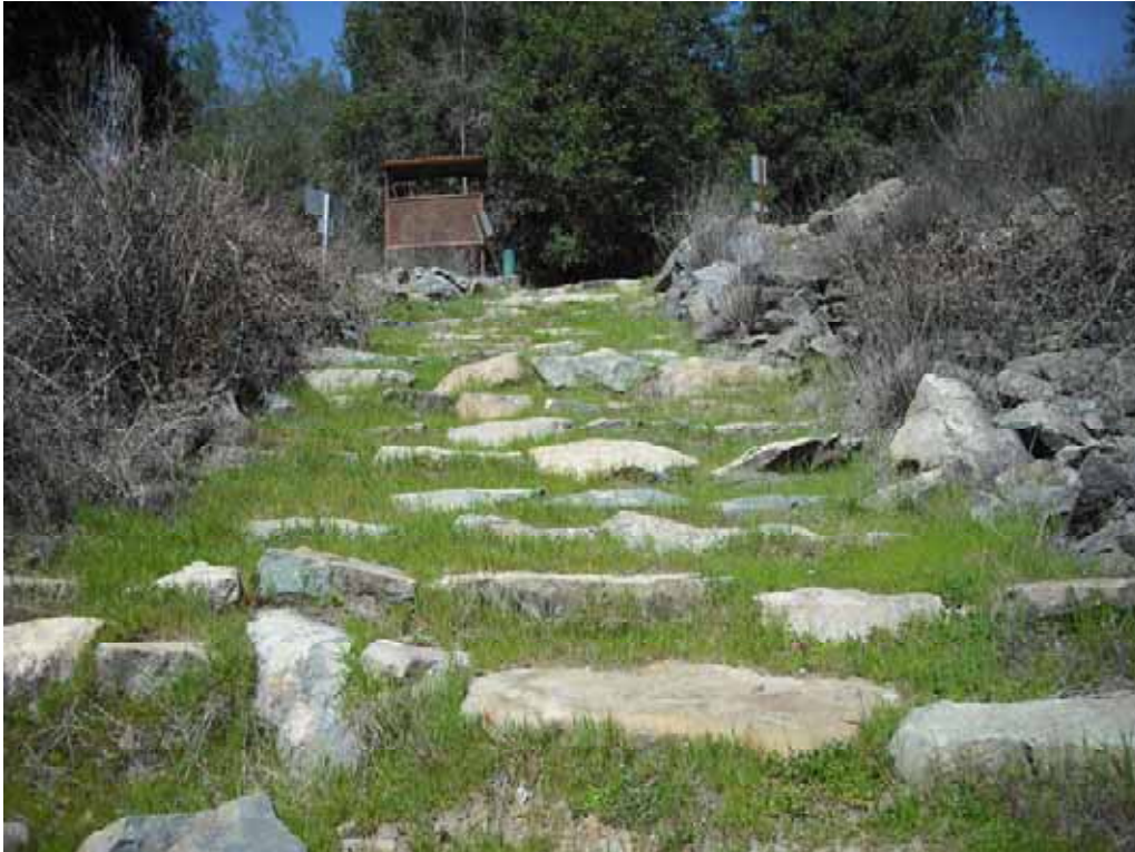
Photo V-2-18. River access stairway located on the south side of the access road across from the Southeast Parking Area. (3/12/09)
