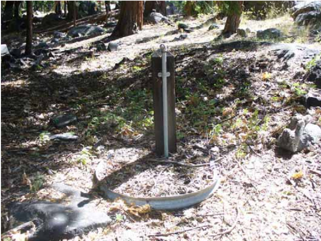
Photo E-2-17. Out of service water faucet. (8/21/09)
