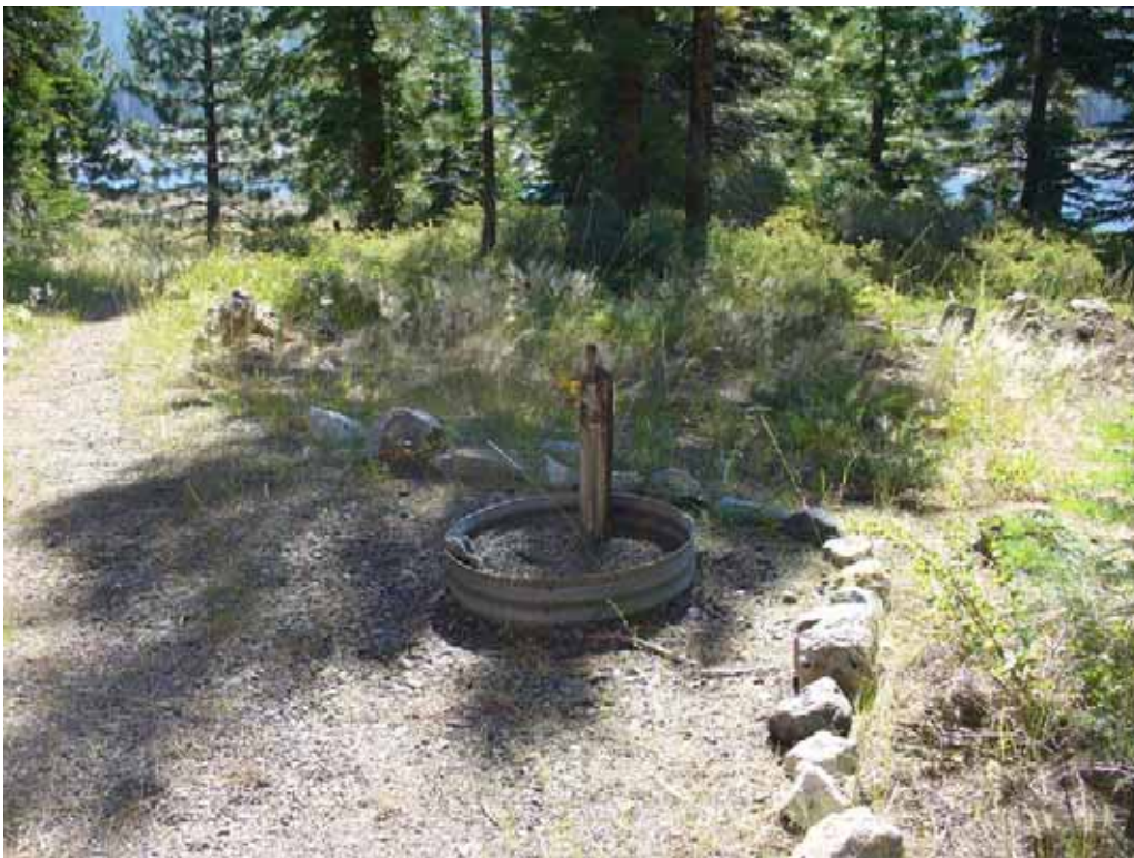
Photo Q-2-12. Water faucet located along path to McGuire Beach, near bathroom. Handle is accessible but approach is not because the sump/drain is set above grade. (7/24/08)
