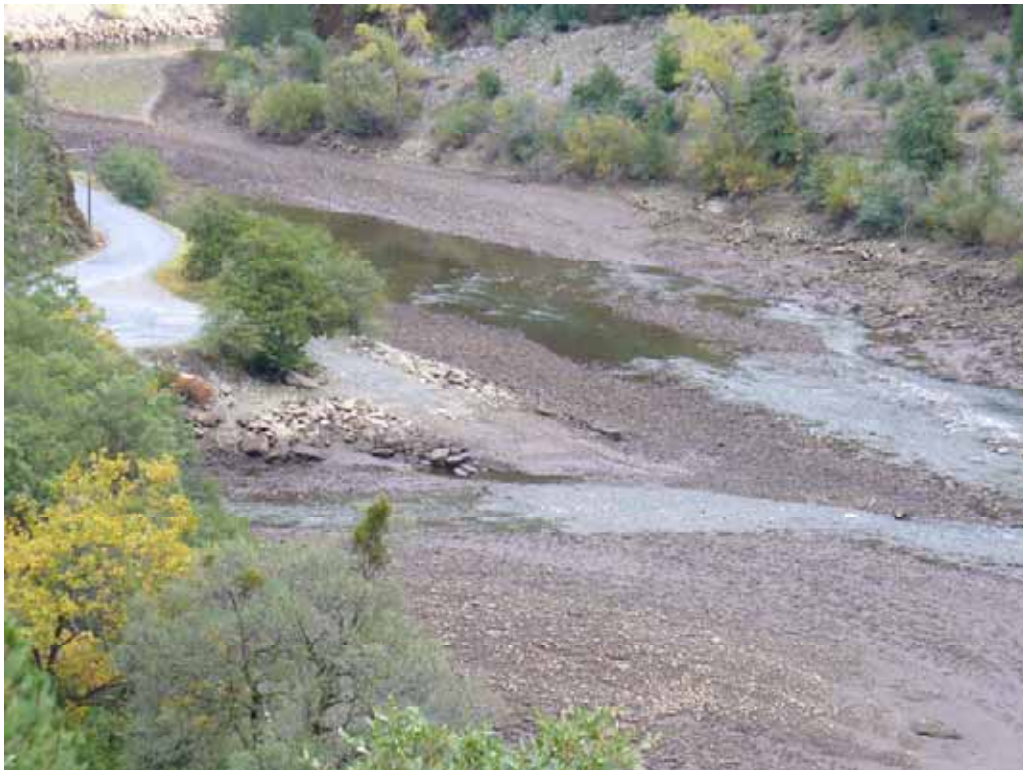
Photo S-2-10. Sediment removal access point on Ralston Afterbay. This site is not a Project recreation facility but is sometimes used to access the reservoir. (11/12/08)
