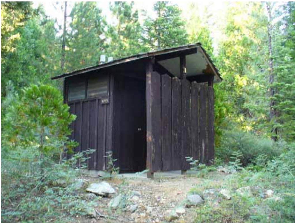
Photo L-2-6. Vault toilet near Poppy Trailhead parking. Not accessible. (7/23/08)
