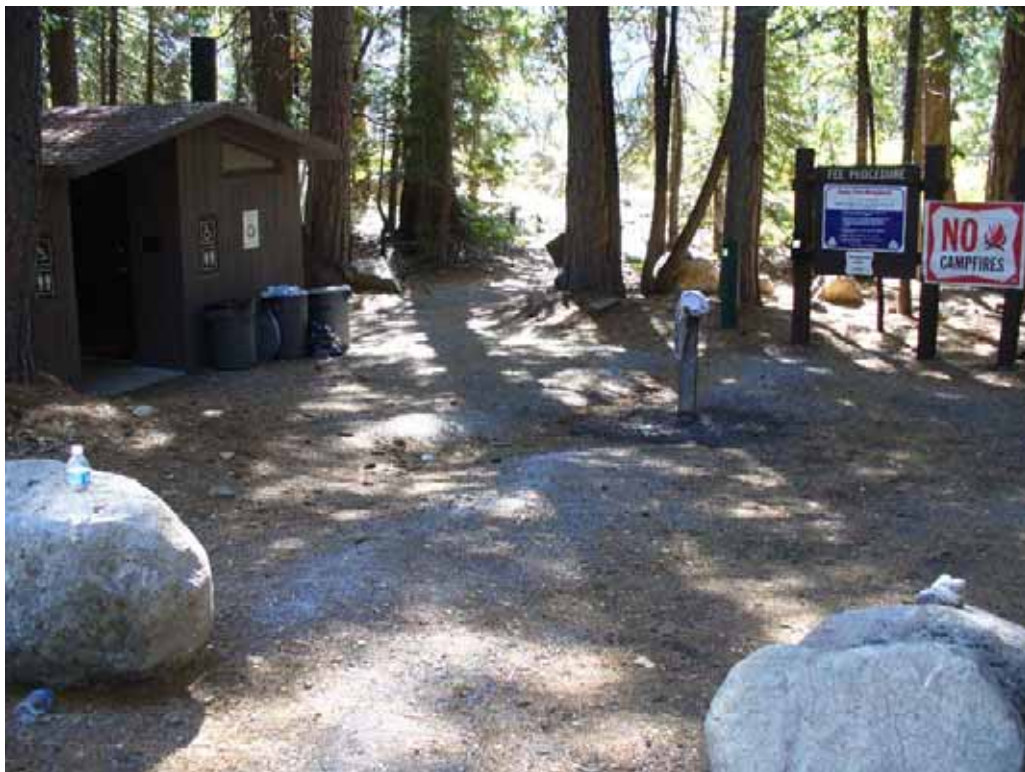
Photo E-2-14. Single unit, accessible, vault toilet adjacent to fee station. Note poor drainage conditions between water faucet and toilet. (8/21/08)
