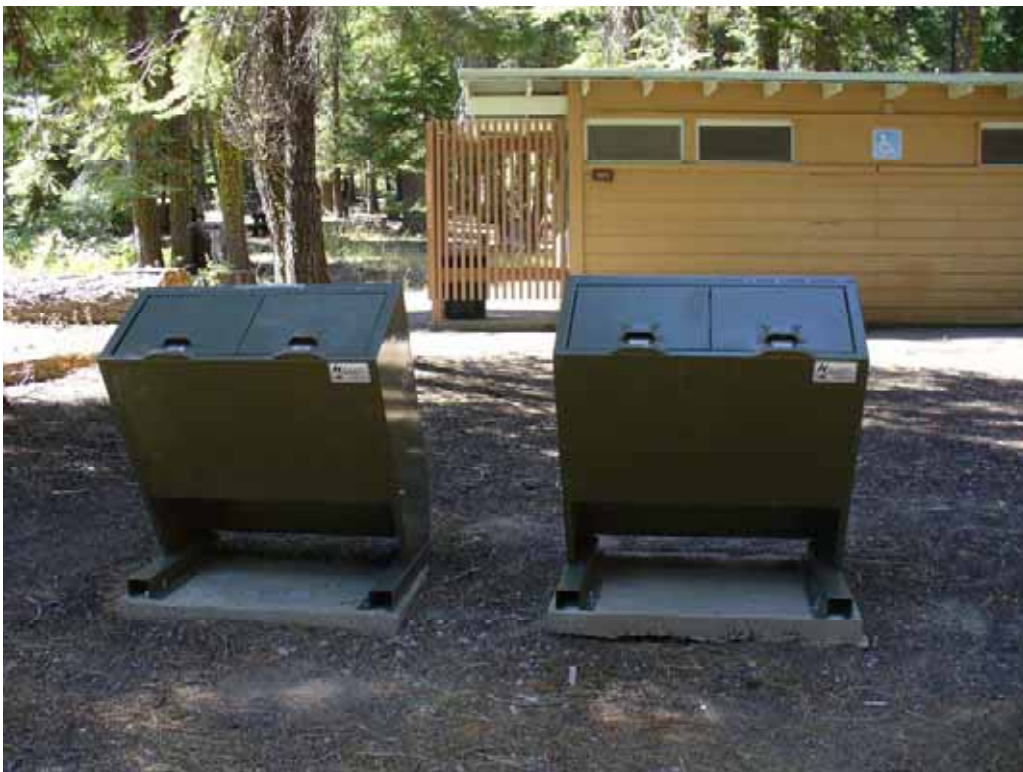
Photo K-2-16. Bear-proof garbage bins on concrete pads. Wood bathroom structure in background has flush toilets and has been converted to meet accessibility standards. (9/04/08)
