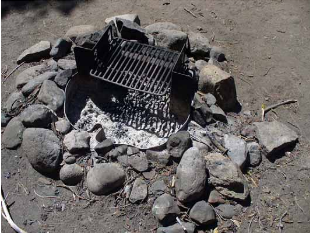
Photo I-2-10. Steel fire ring and grill, poor condition. (9/04/08)
