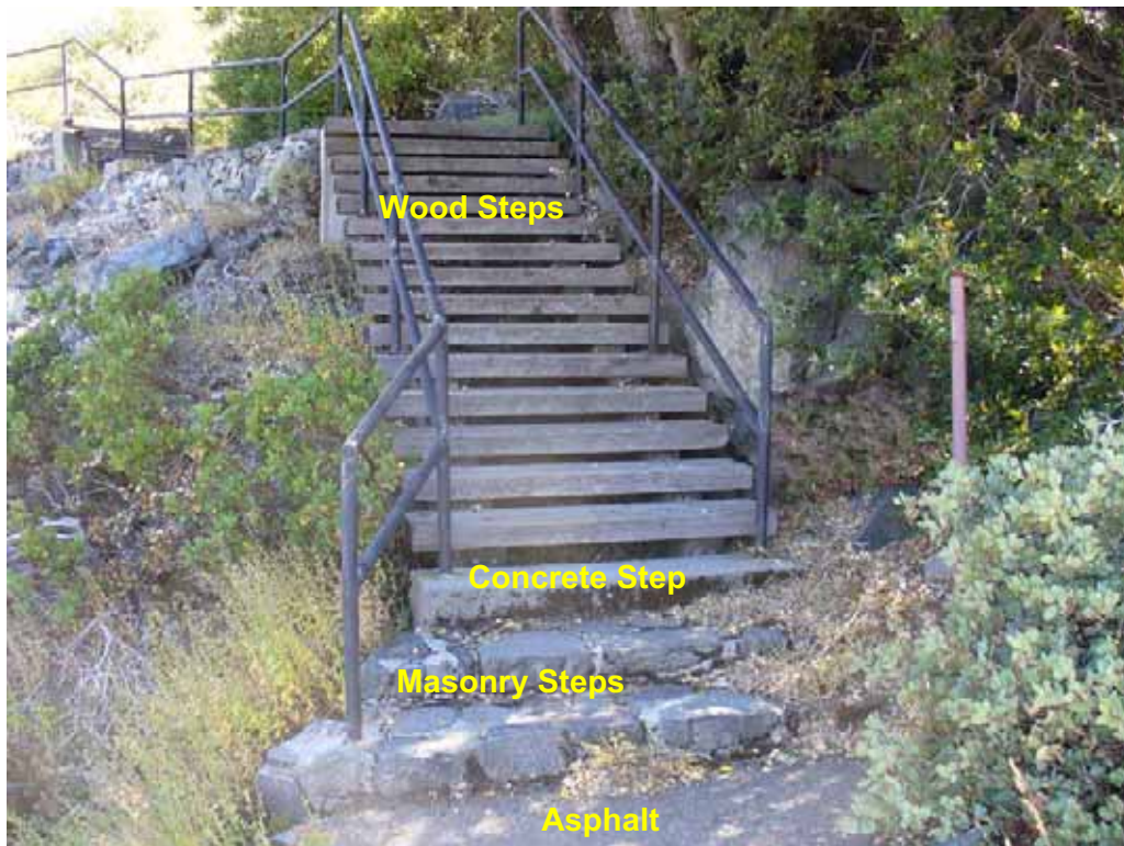
Photo H-2-32. Lower portion of trail/stairway looking up towards General Parking Area. Note various surface types: asphalt landing masonry steps/concrete step/wood steps. Also note steel handrails. Not disabled accessible. (8/4/08)
