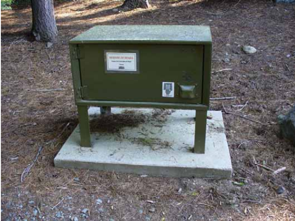
Photo J-2-18. Typical bear-proof food storage locker (bear box) on concrete pad. (7/24/08)
