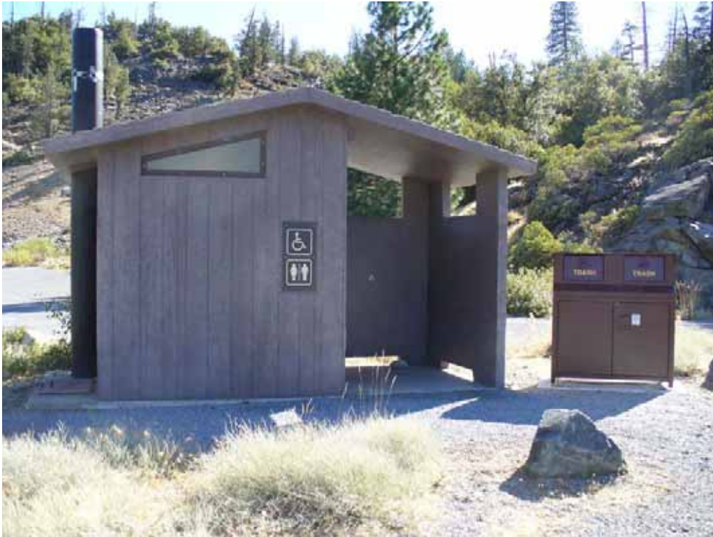
Photo H-2-23. Single unit pre-cast concrete toilet (CXT) located in Hell Hole Boat Ramp General Parking Area. Restroom is disabled accessible and in good condition. Note bear-proof garbage container adjacent to restroom. (8/4/08)
