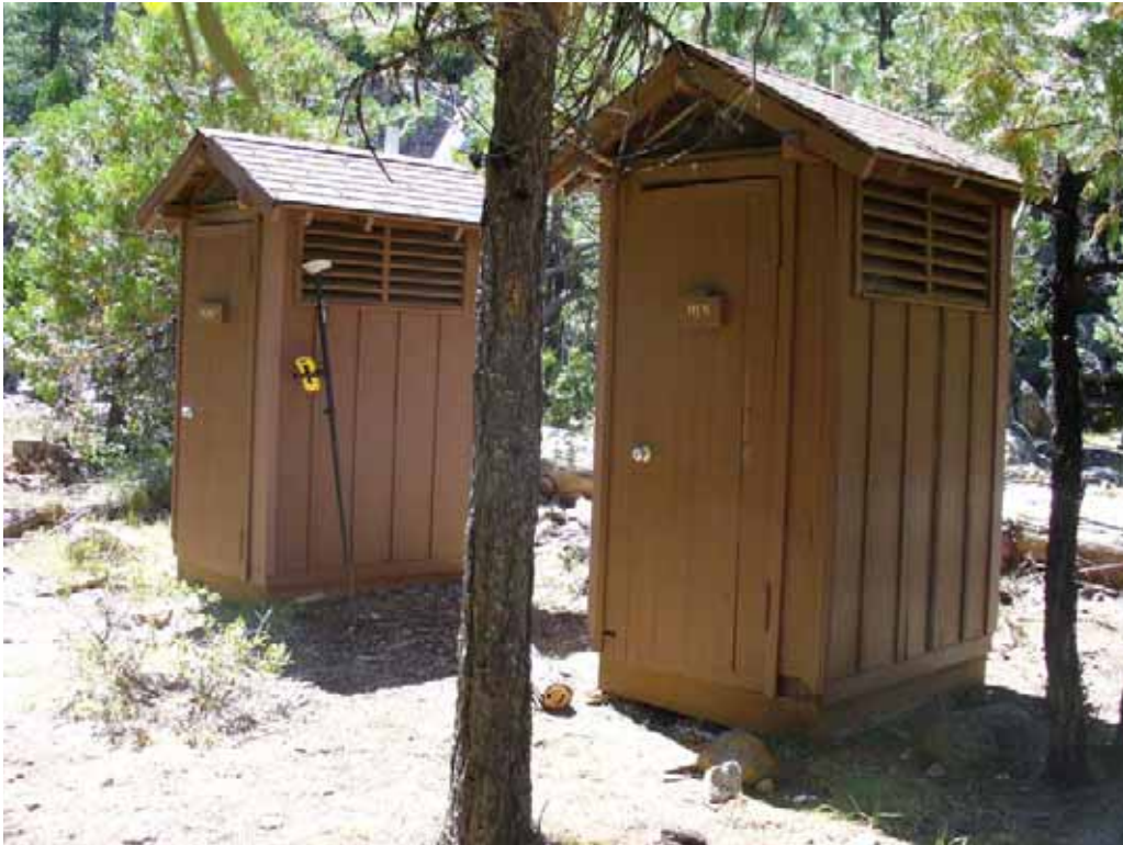
Photo F-2-1. Pit toilets 1 and 2. (8/4/08)
