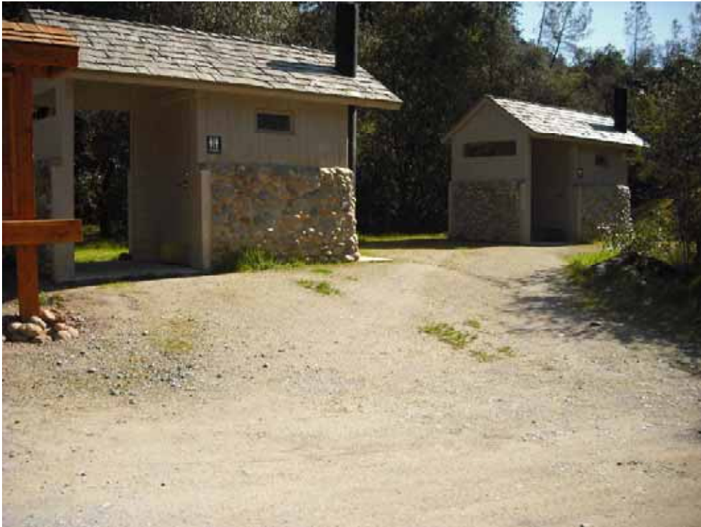
Photo V-2-3. Two coed bathrooms located in Northwest Parking Area. Disabled accessible and in good condition. (3/12/09)
