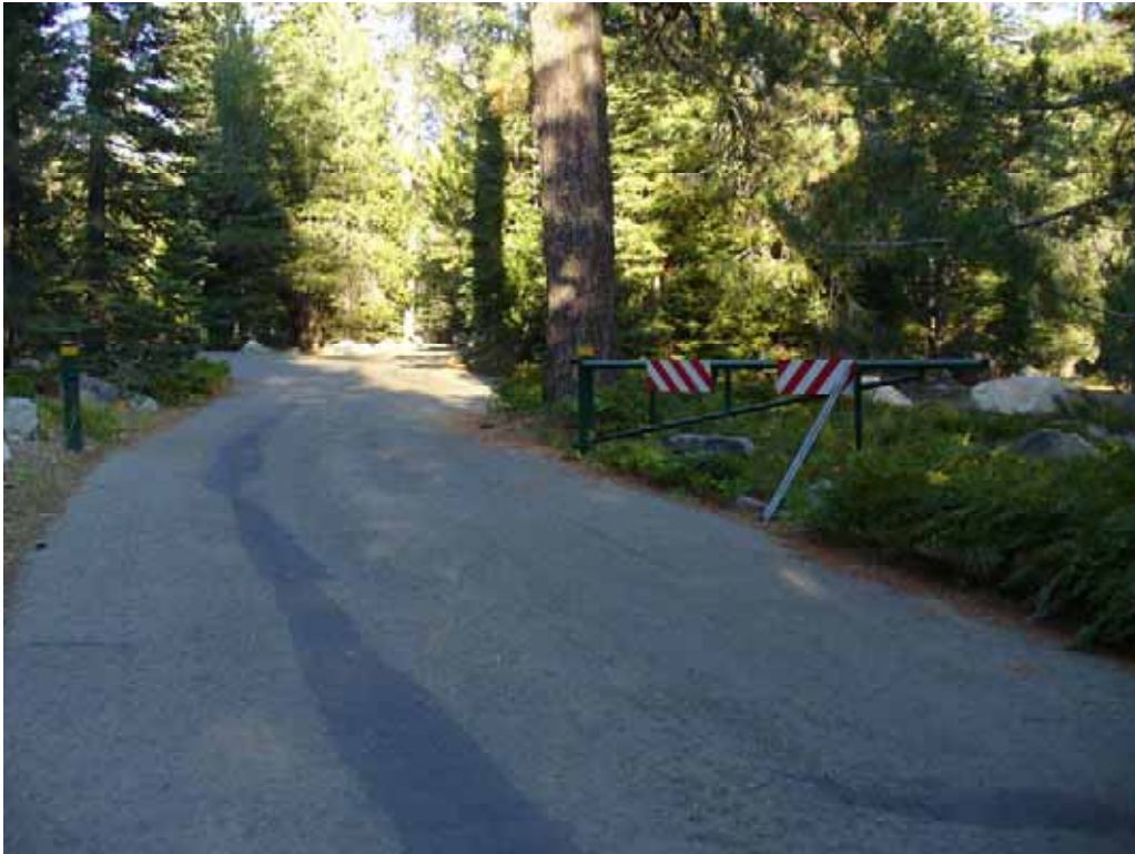
Photo N-2-5. Swing gate along main access road near Aspen, looking north towards Lodgepole. This gate was installed in September 2006. (7/23/08)
