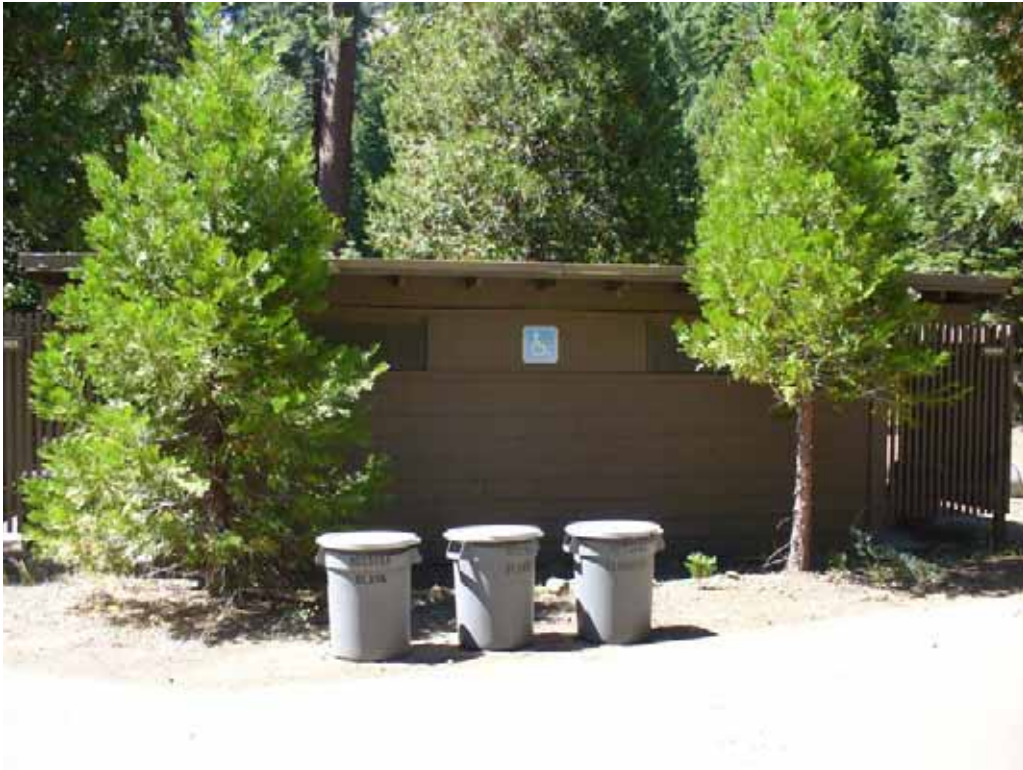
Photo D-2-11. Bathroom with flush toilets located near Site 52. This bathroom was converted to be accessible by PCWA in 1995. (8/21/08)
