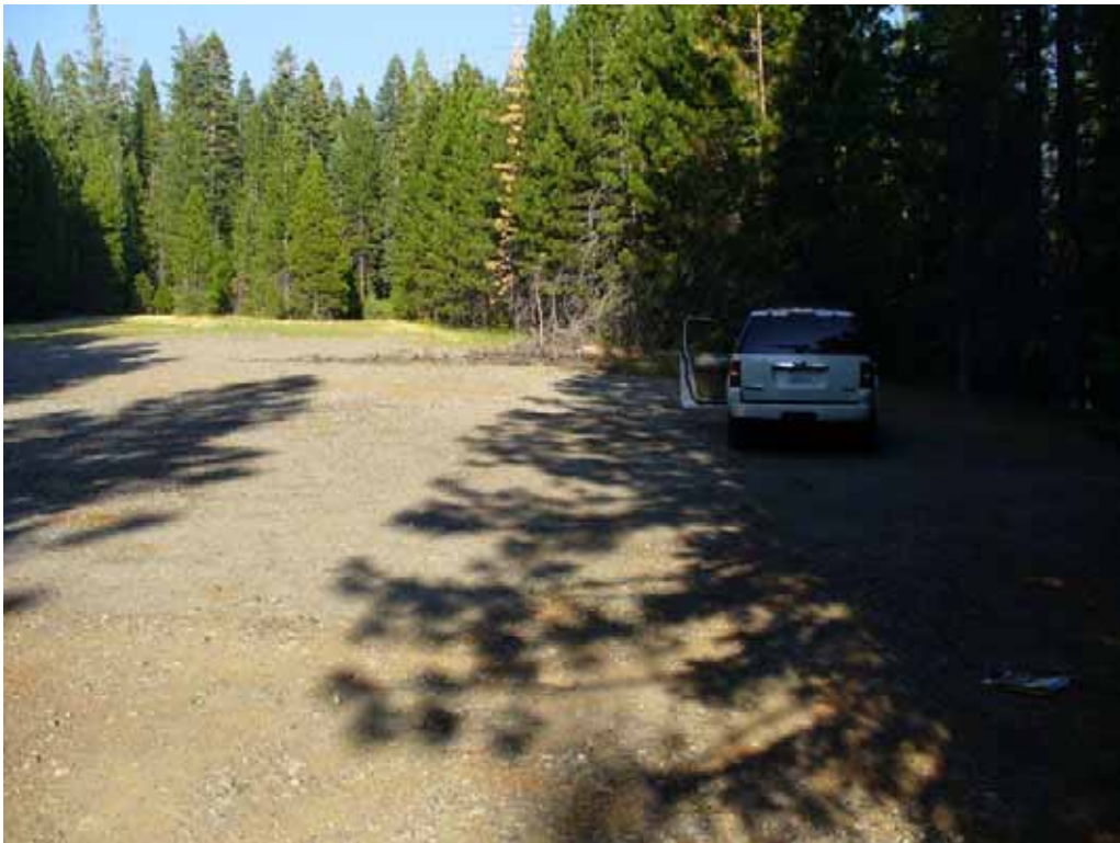
Photo P-2-6. McGuire Boat Ramp Parking Area – southeast lot. Surface has deteriorated to base rock and is in poor condition. (7/23/08)
